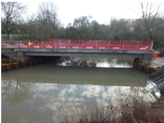
Figure 2 Photograph of bridge from temporary bridge
