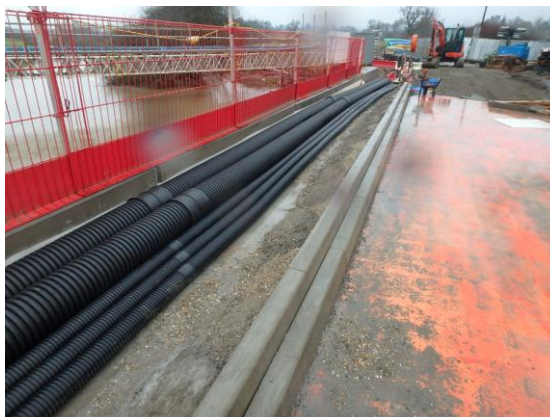
Figure 1 Photograph of ducting for pipes and new kerbs
