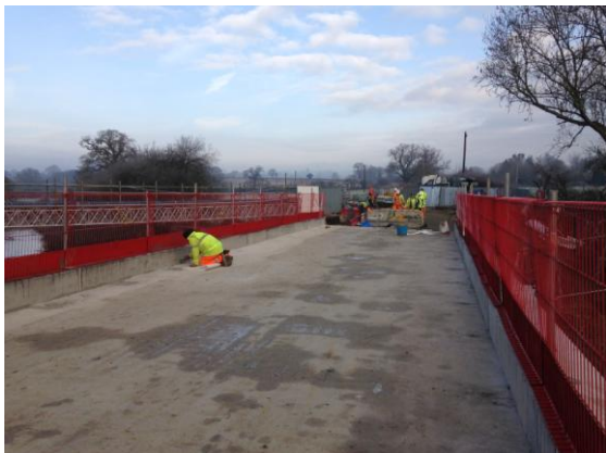
Figure 4 Photograph of concrete bridge deck
