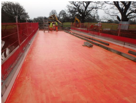
Figure 3 Photograph of waterproofing on bridge deck
