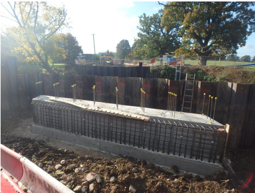
Photographs showing newly constructed concrete abutment and auger used to construct the concrete foundation piles on the south side of the river.
