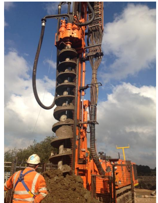
Photographs showing newly constructed concrete abutment and auger used to construct the concrete foundation piles on the south side of the river.
